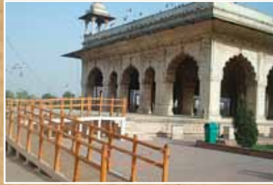
Ramps at Red Fort, a World Heritage Site
