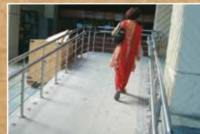
Ramp at NDMC Building - post implementation of Svayam's Audit Report
